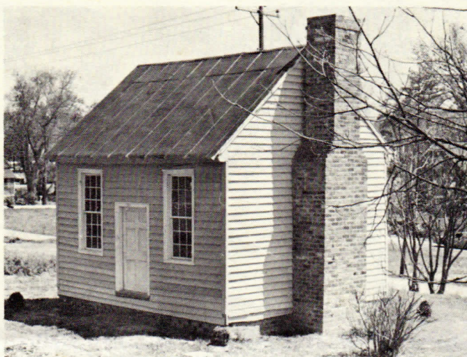
Taken before renovation was completed, this photograph shows the west side of the Manly Law Office before steps or shutters were in place.
