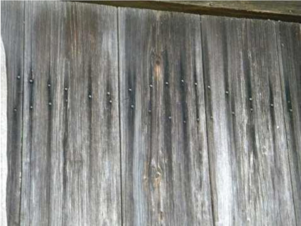
Smokehouse door detail, 2014. Photo by Beverly Wiggins
