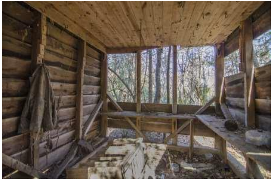
Smokehouse dropped ceiling and interior detail. Photo by Duane Hall.
