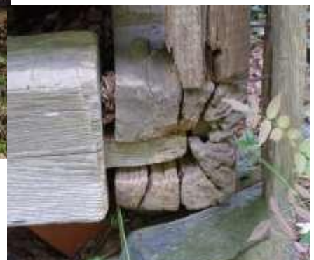
Smokehouse sill detail. Photo by Barbara Pugh.
