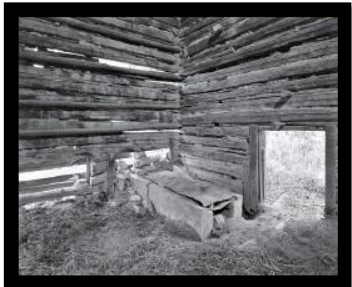
Figure 7. A typical furnace inside an abandoned barn
