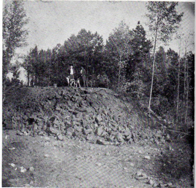
Site of railroad during construction, about 1888.
