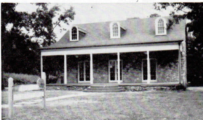
The Community House, half a block east of Hillsboro Street on Thompson Street, was built in 1936, funded by the W.P.A. as a make-work project during the Depression. It was renovated in 1985 to restore its original appearance.
