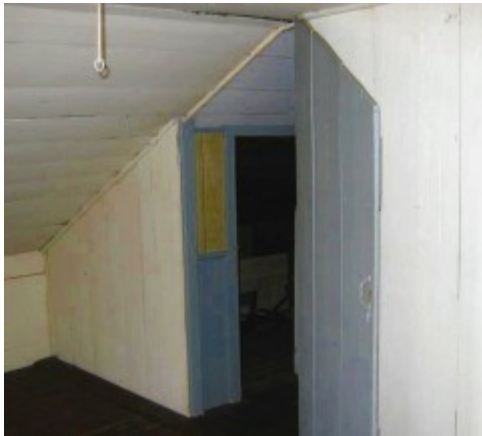
Door into southeast room
