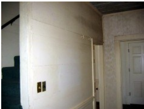
Sheathed hall and stairs
