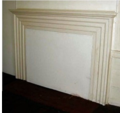
Sealed fireplace in upstairs west room
