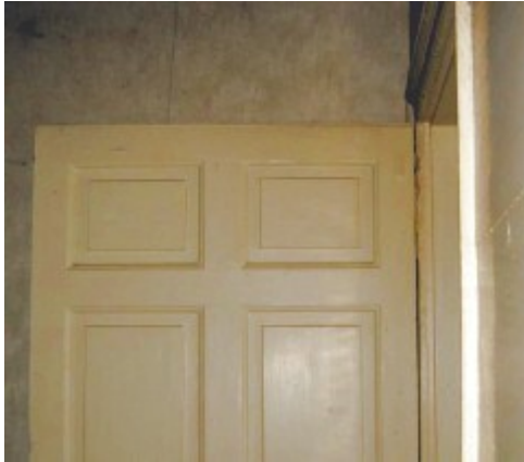
Six-panel door in hall
