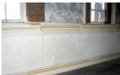
Windowsill and molding 2006
