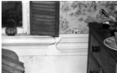
Windowsill and molding 1975*
